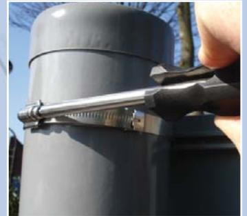
Screw the band through using a hand or power tool.
