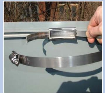
Thread the band through the slots in the sign and around the post.
