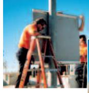
This 4' x 4' .080 gauge aluminum sign was installed in less than 5 minutes using SIGNFIX Large Corner Angle Channel Extrusion and
